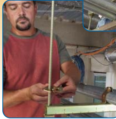
Standard installation requires manual threading of bolt on threaded rod.
