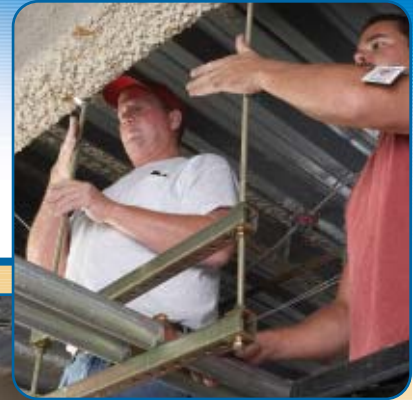
Standard installation requires manual threading of bolt on threaded rod.
