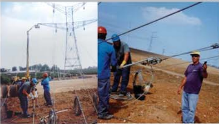
CONTROLLED CABLE TENSIONING
