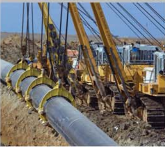
GAS PIPELINE INSTALLATION
