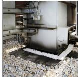
Our low-profile flat sock for oils and fuels but not water provides more ground contact for the best protection against seepage.
