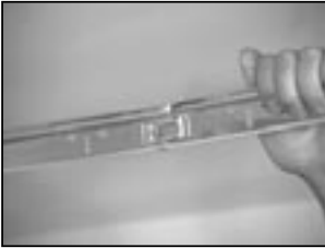
Join sections of main beam
