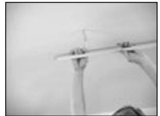
Install first main beam
