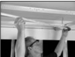
Square the grid by measuring across the diagonal of the grid opening
