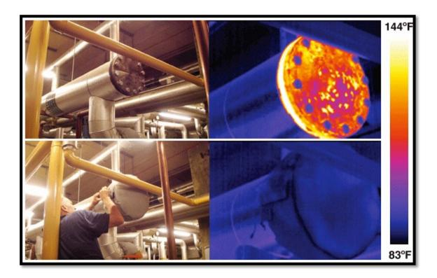
UniTherm's removable insulation jackets are an effective and convenient way to prevent heat loss, and protect equipment and personnel. UniTherm insulation jackets are designed with draw cords and lacing hook and wire. This makes them easy to install, remove, and reinstall.
