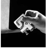
1. Position hanger on C or Z purlin or on horizontal flange. (Z purlin shown)
