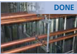
Level, tighten lock nut
