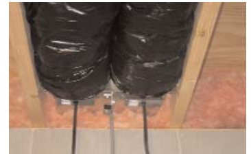
Install 6" rigid, flexible or insulated flexible duct on DT2-6 take off. Firmly secure duct to take off with included zip ties. Insulated flex should be used in cold climates where supply air is brought in to prevent condensation. Properly support duct to minimize sagging, bends and sharp turns that may restrict air flow.
