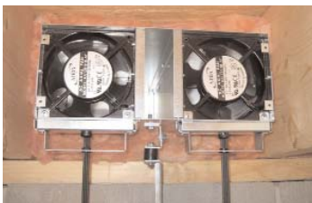
Remove (4) screws and remove rear plate from XCHANGER™.
