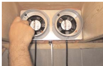
Install DT2-6 on rear of XCHANGER™ with (4) screws removed previously.
