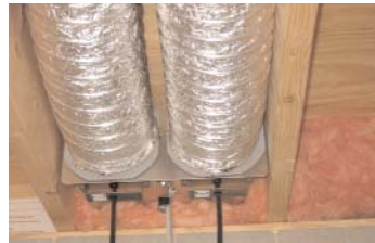
Install 6" rigid, flexible or insulated flexible duct on DT2-6 take off. Firmly secure duct to take off with included zip ties. Insulated flex should be used in cold climates where supply air is brought in to prevent condensation. Properly support duct to minimize sagging, bends and sharp turns that may restrict air flow.
