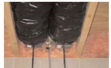
Install 6" rigid, flexible or insulated flexible duct on DT2-6 take off. Firmly secure duct to take off with included zip ties. Insulated flex should be used in cold climates where supply air is brought in to prevent condensation. Properly support duct to minimize sagging, bends and sharp turns that may restrict air flow.
