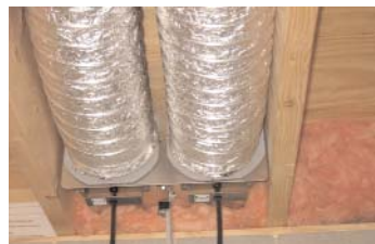
Install 6" rigid, flexible or insulated flexible duct on DT2-6 take off. Firmly secure duct to take off with included zip ties. Insulated flex should be used in cold climates where supply air is brought in to prevent condensation. Properly support duct to minimize sagging, bends and sharp turns that may restrict air flow.
