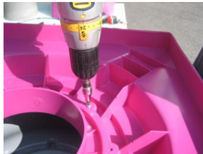
11. Screw the roof curb cap to the housing.
