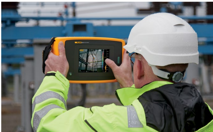
Image taken of the ii910 Precision Acoustic Imager detecting partial discharge in a high voltage application.
