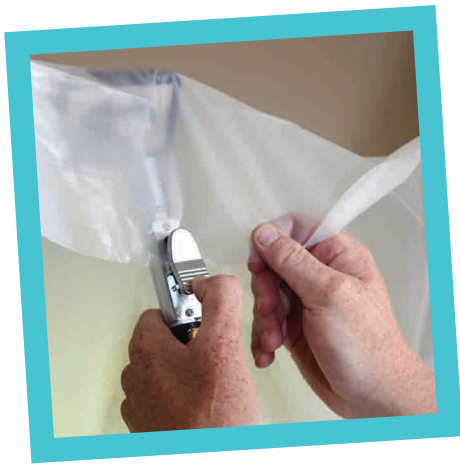
clip plastic onto quick clip
