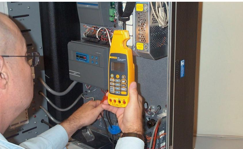
Checking communication wiring voltages on automation system controls.
