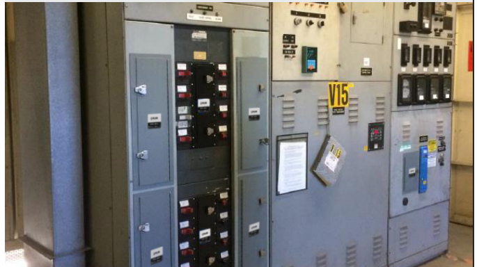
Figure 1: Final installation of the IR windows
