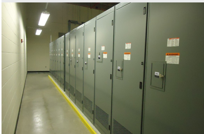
Figure 3: Finished installation of IR windows
