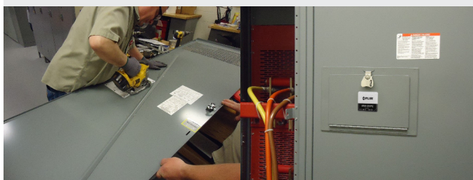
Figure 1: Field Installation of IR windows using provided templates and a jigsaw
