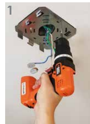
1 Mount plate to junction box.
