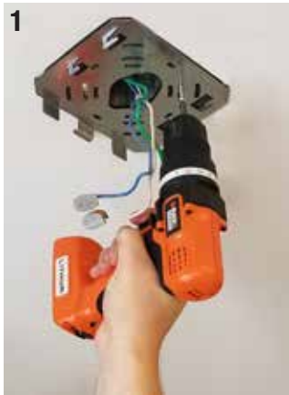
Mount plate to junction box.
