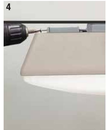
Two mounting screws close and secure fixture to the mounting bracket.
