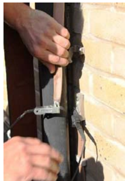
Two pole test
