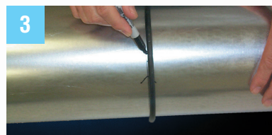
Use O-ring provided and mark for cut.
