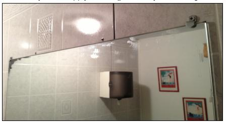
**2.** Re-locate Z-Clips to edges of mirror approx. 1 inch in from the edge of mirror.
