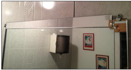
**3.** Apply Vertical Acrylic Mirror Framing Strips to sides of mirror up to the Z-Clips. Then apply Horizontal Framing Strip in between vertical strips and even with the top of the Z-Clips.
