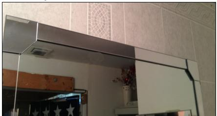
**4.** Apply Acrylic Mirror Corner Plates in corner areas on top of Acrylic Mirror Strips where the vertical and horizontal framing strips meet in each corner which covers the Z-Clips!
