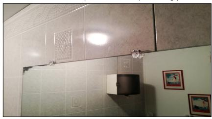
**1**. You will need to replace the standard plastic mirror clips with thin metal "Z-Clip" Mirror Clips.
