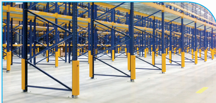
Schneider Electronics new warehouse full installation - (France).
