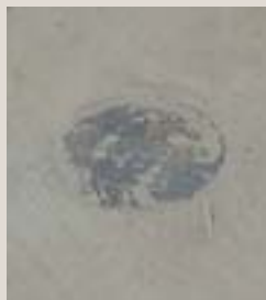
6. Finished concrete over device
