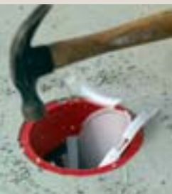
7. Break and remove cap
