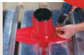
Deck Adaptor works great on uneven surfaces like fluted steel pan decks
