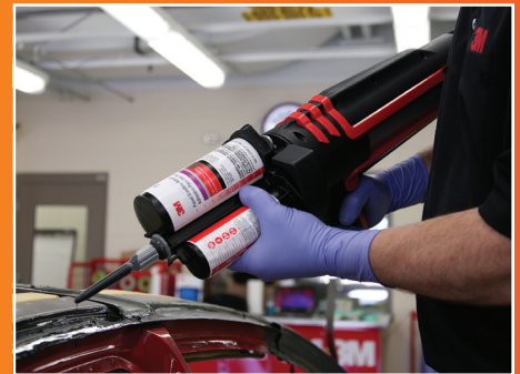
Roof Panel Bonding
