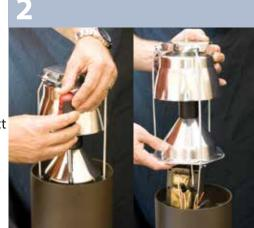
Insert LED retrofit unit and connect wires, tighten three mounting screws
