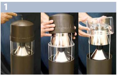
three mounting screws, lift out existing unit and disconnect wires
