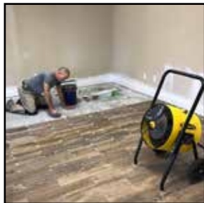
Pole Building / Workshop
