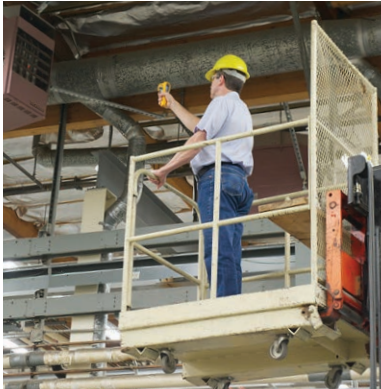
Identifying the temperature of ceiling-mount equipment.
