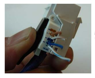
**Step 4.** Use the included lever to snap the lid all the way down.
