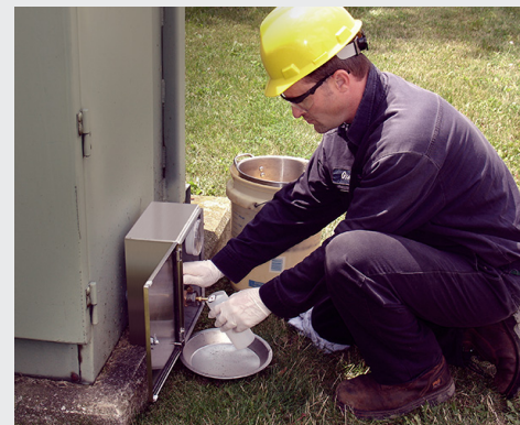
External Oil Sampling – Courtesy of SDMyers
